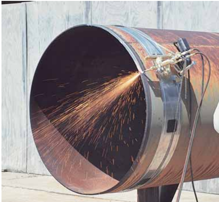
Cutting 48" pipe with Band-Type Pipe Beveler
